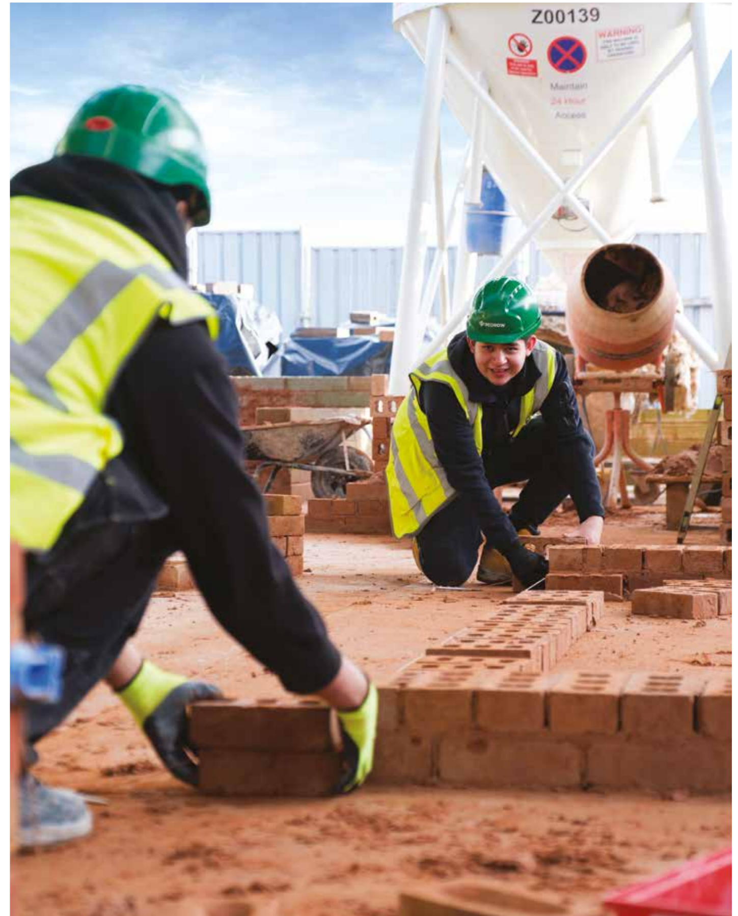
Bricklaying apprentices at the NHBC Training Centre, Tamworth.
