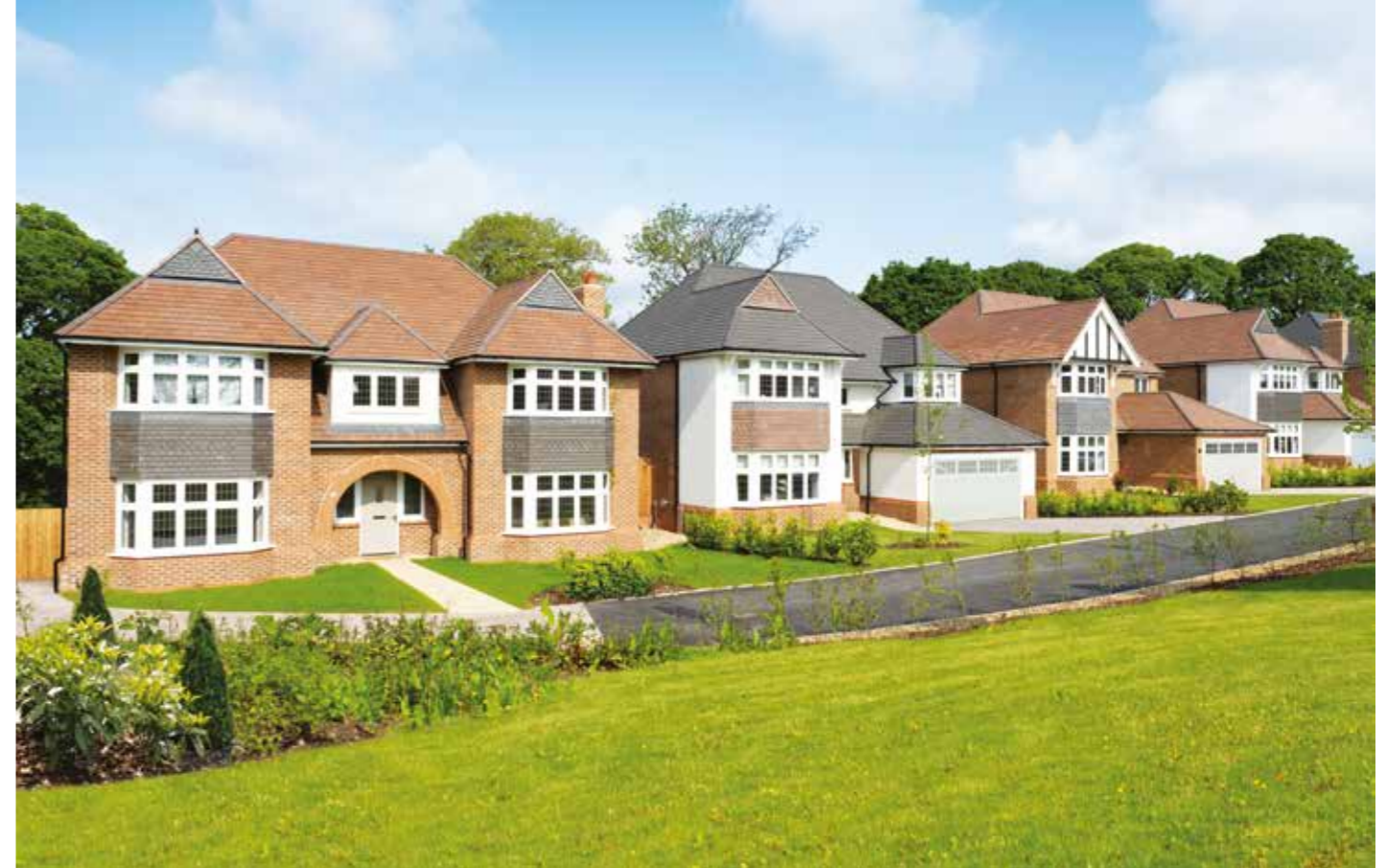
↑ Sycamore Manor, Chorley, Lancashire.
