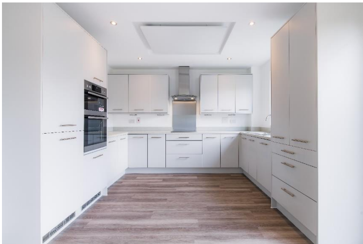
Figure 1: Ceiling Installation of IR panels
