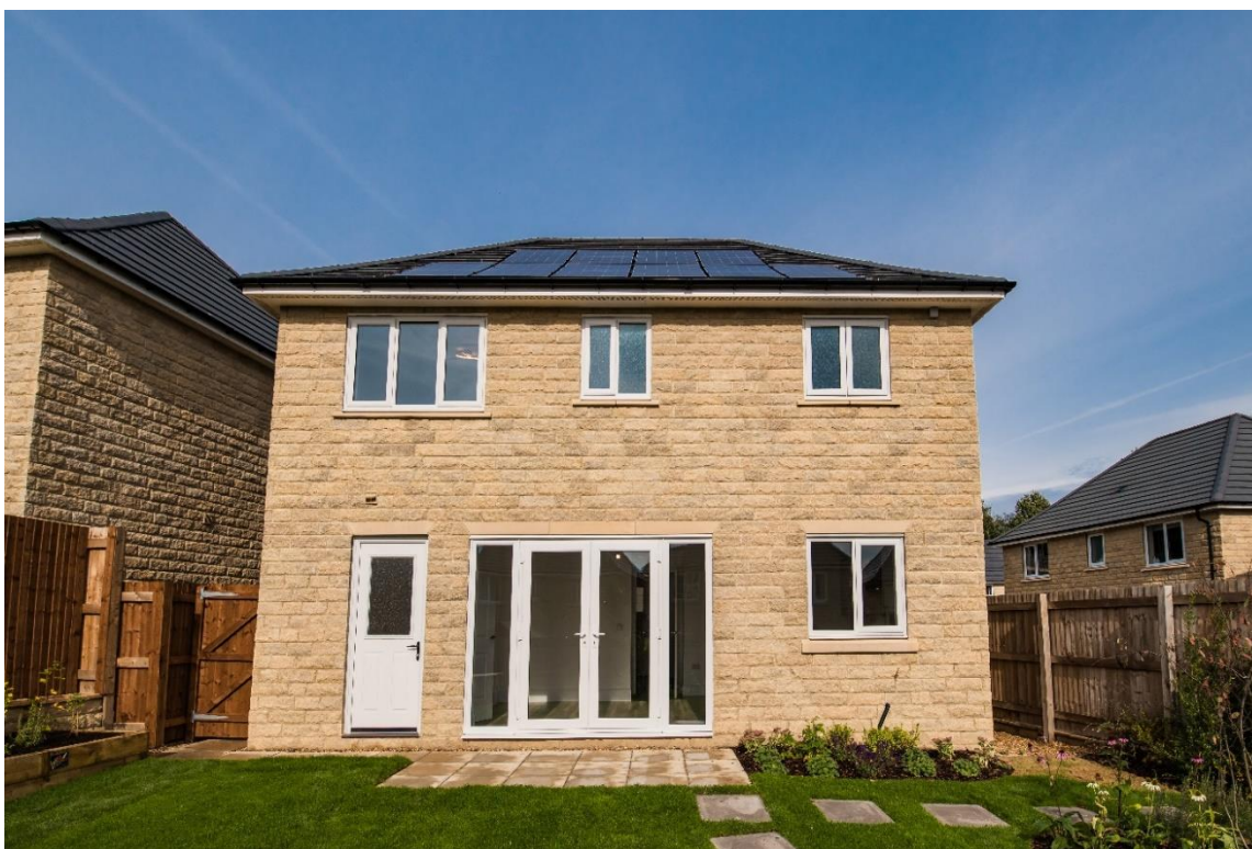
Figure 3: Photograph showing PV installation.
